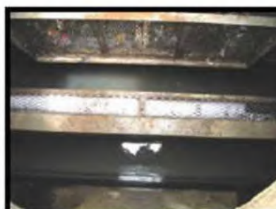
Remove Old Hydrocarbon Booms & Replace with New Ones.
