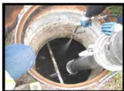
If Sediments are Compacted Use a Pressure Washer to Loosen Up Sediments.
