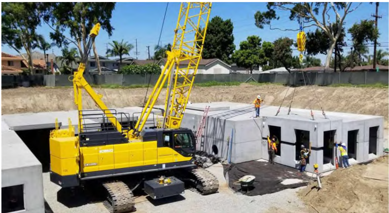
Figure 5-8. Precast units being installed at Caruthers Park, Bellflower
