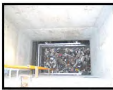
Assess Condition and Pollutant Loading Through Visual Inspection. Look at Trash & Sediment Loading.
