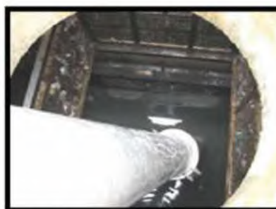
Open Screen Panels & Insert Hose into First Separation Chamber to Remove Sediments. Repeat in All Three Chambers.
