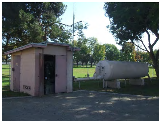
Figure A-42 Well #6 and Hydropneumatic Tank
