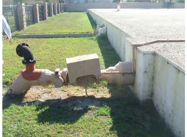
Figure A-28 Plant 22, Altitude Valve
