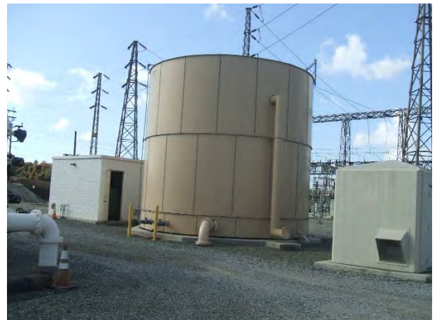
Figure A-12 Plant 4, Arsenic Backwash Tank
