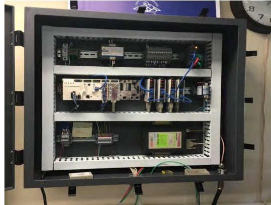
Master Telemetry Panel
