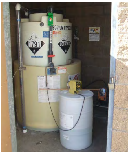
Figure A-37 Well #15A Chlorination
