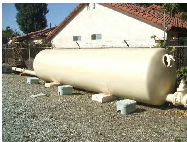
Figure A-41 Well #18 Hydropneumatic Tank
