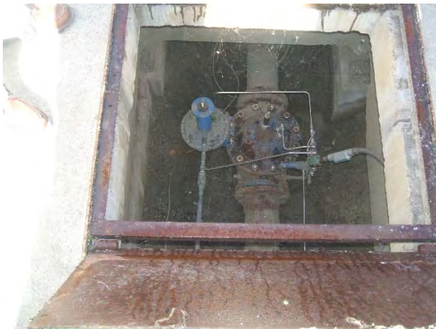
Figure A-20 Plant 13, Altitude Valve
