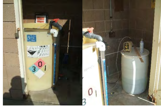
Figure A-34 Well #10 Chlorination
