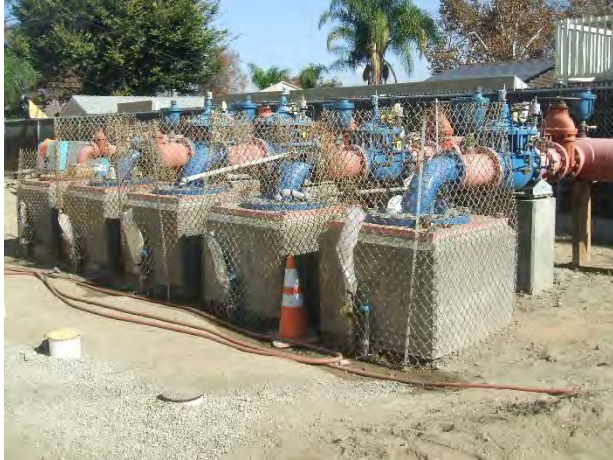
Figure A-19 Plant 13, Booster Pumps #1, #2, #3, and #4
