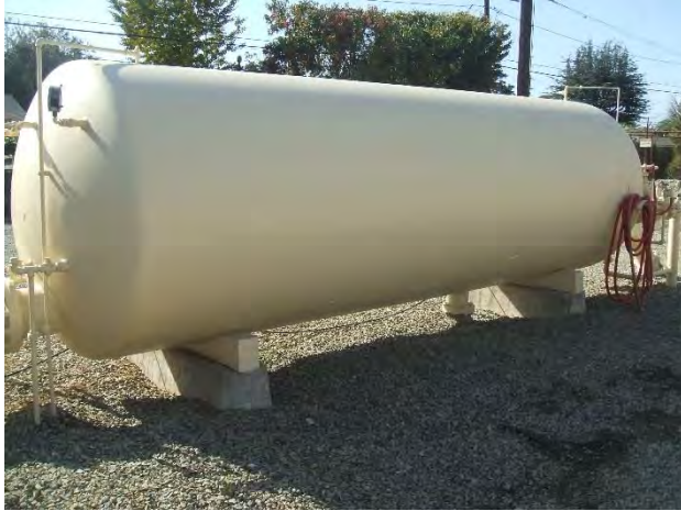
Figure A-7 Plant 4, Well #4 Hydropneumatic Tank
