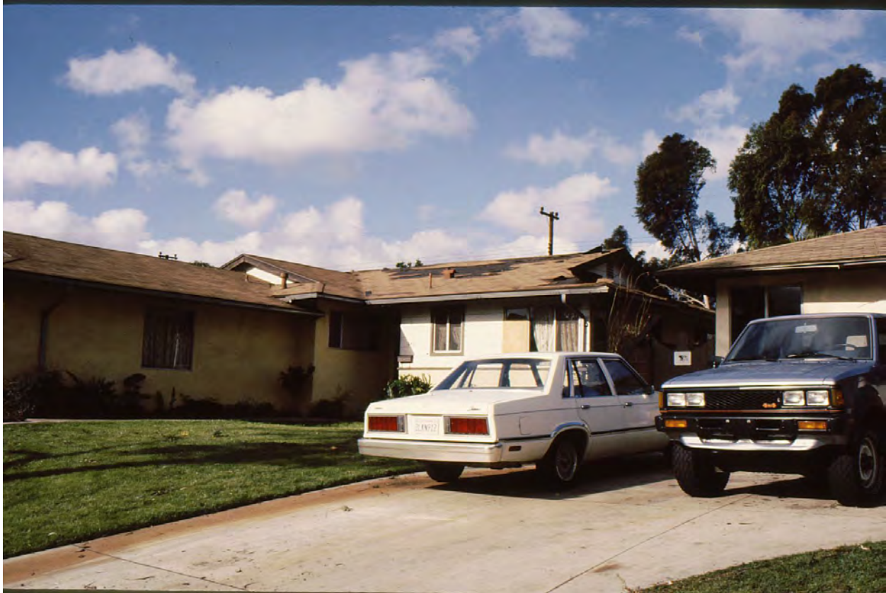
Figure 8-3: Roof Damage from 1991 “Mini-Tornado”
