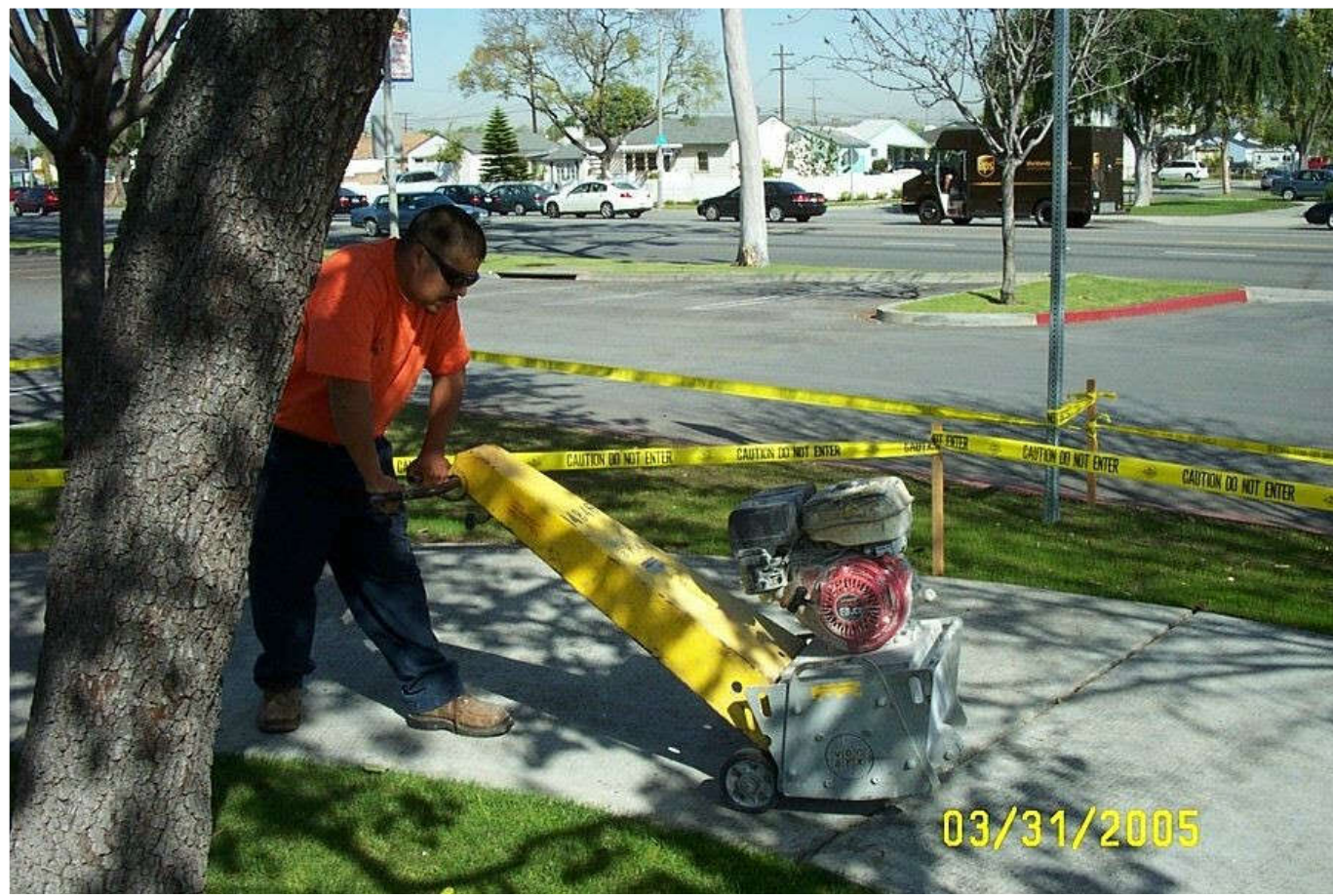
Sidewalk Grinding
