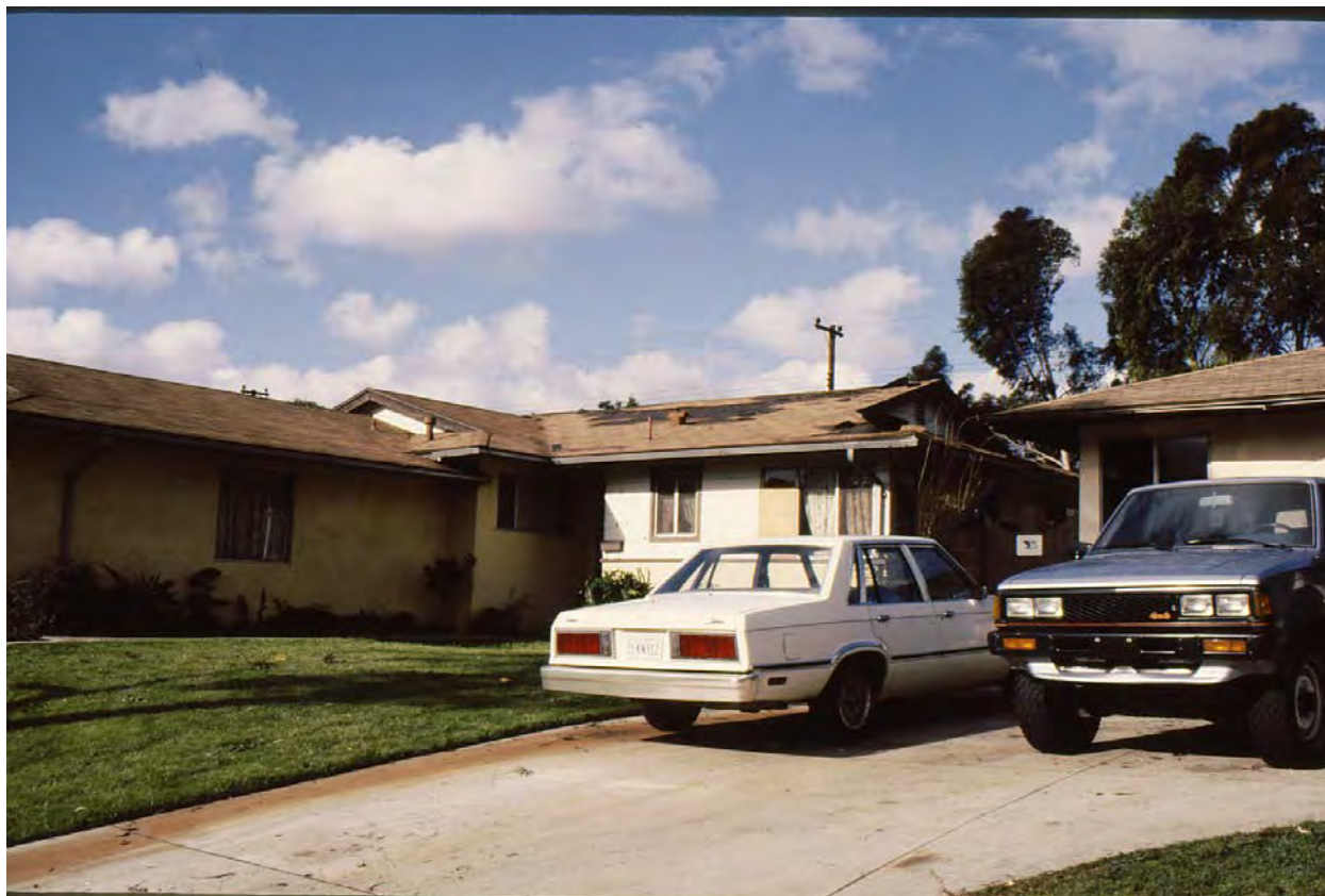
Figure 8-3: Roof Damage from 1991 “Mini-Tornado”
