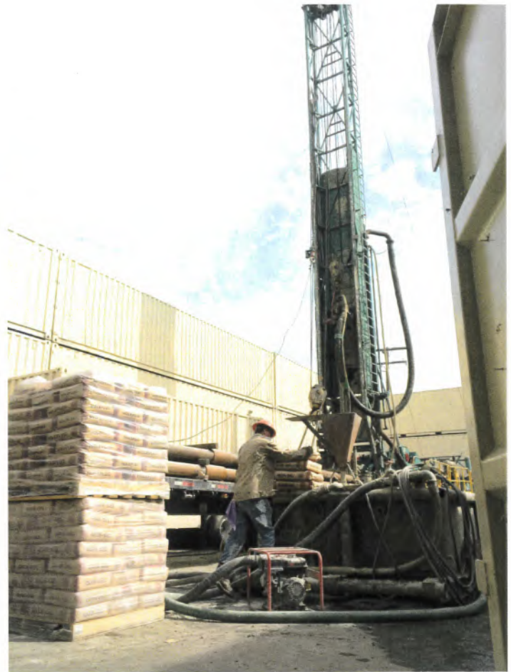
Our field staff will collect and log geologic samples during pilot borehole drilling to determine locations for zone isolated aquifer zone testing
